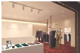
Retail shop Lighting
